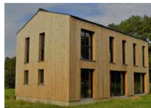
A la pose
