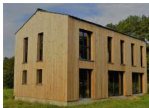
A la pose
