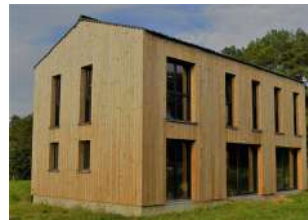
A la pose
